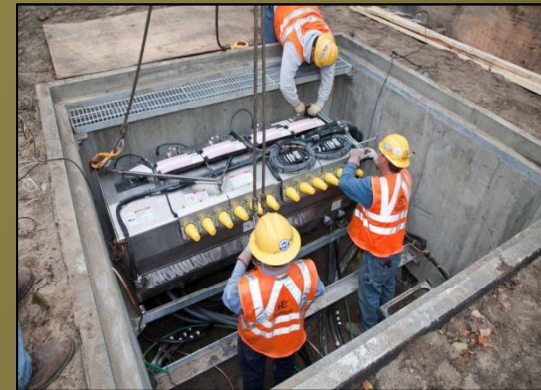
Specially configured Remote Supervisory Vista Underground Distribution Switchgear
