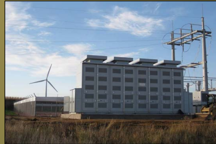
Luverne, Minnesota NaS Battery Installation
