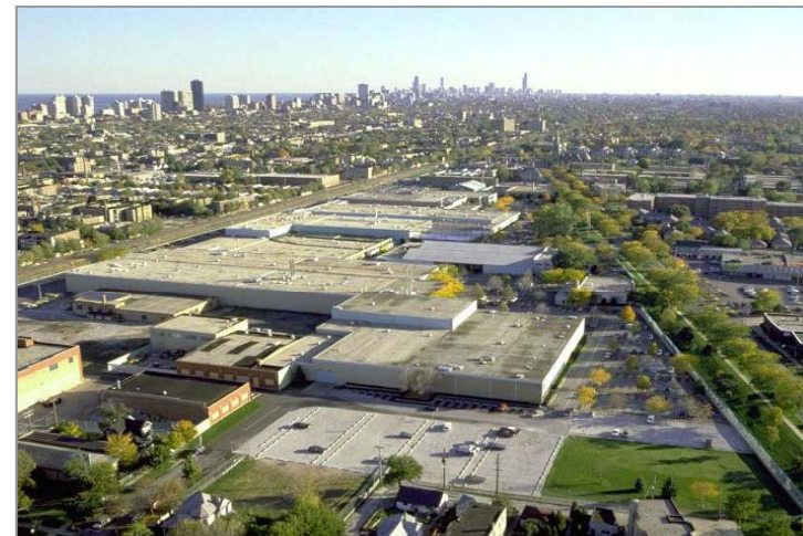
S&C Electric Company John R. Conrad Industrial Campus Chicago, Illinois
