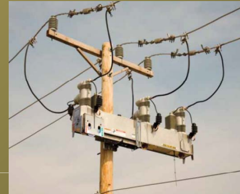
IntelliRupter Self Powered, Self Contained, Fault- Interrupting Switch
